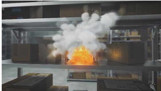
3. The fuse cords running along the surface of the housing activate the spray cartridge inside the device
