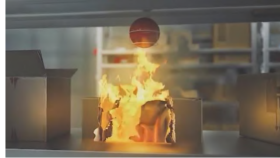
2. Fire comes in contact with the "FINFIRE" device.
